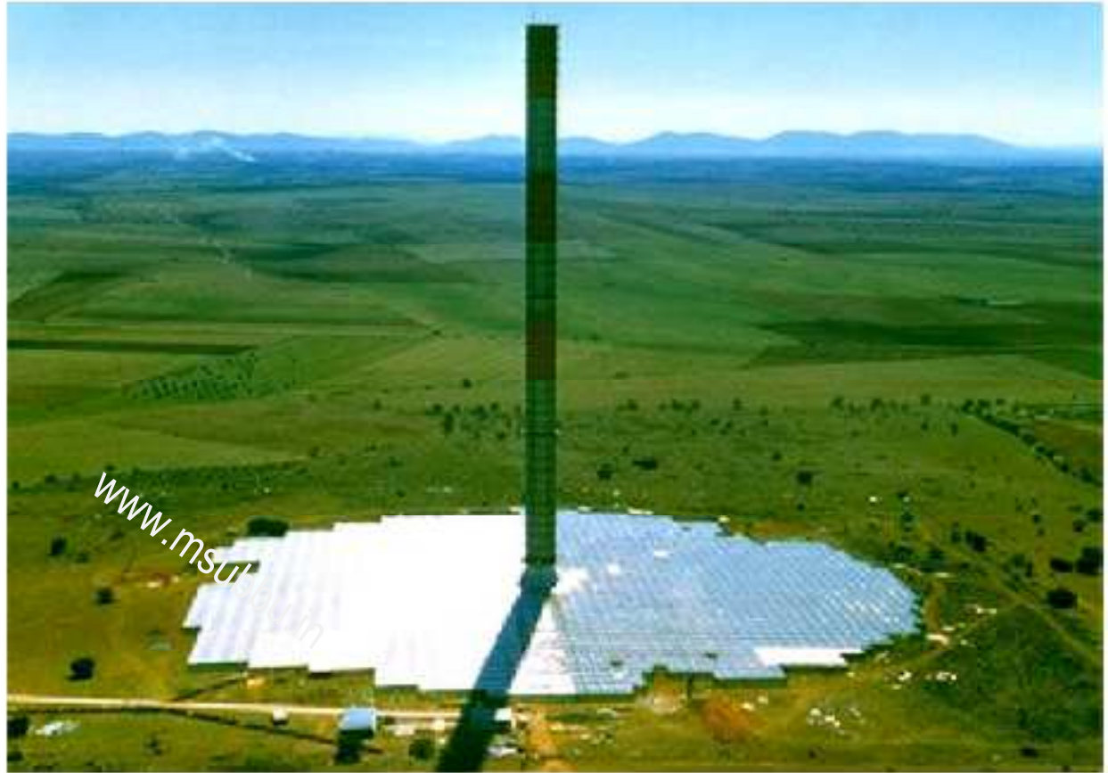
Figure 6 50 kW Solar chimney pilot project , Manzanares, Spain
