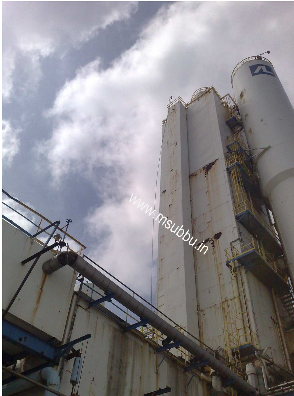
Liquid Air cold box (Distillation Column). Its exterior is basically a metal casing stuffed with insulating materials such as wool
