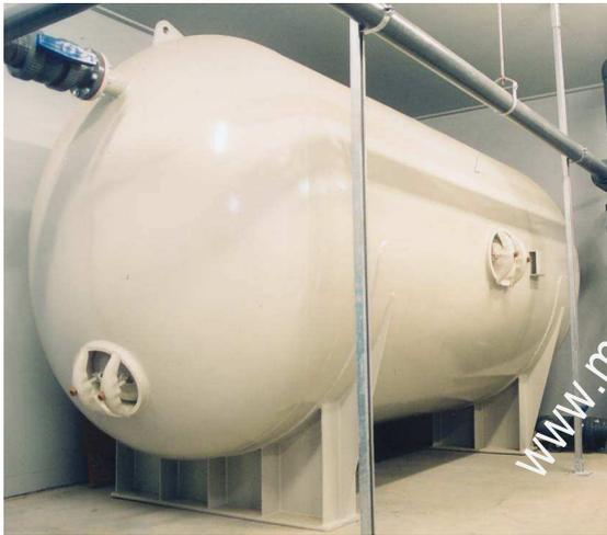
In selecting the location of the saddle supports it is preferable to make dimension  $A$  less than  $R$  in order to take advantage of the head. Dimension  $A$  is often selected so that  $A = 0.4R$ . Dimension  $A$  should never exceed 20% of dimension  $L$ ; otherwise the stresses resulting from cantilever action will be excessive. Horizontal pressure vessels are generally fixed at one saddle and the other is allowed to move to accommodate thermal expansion.
