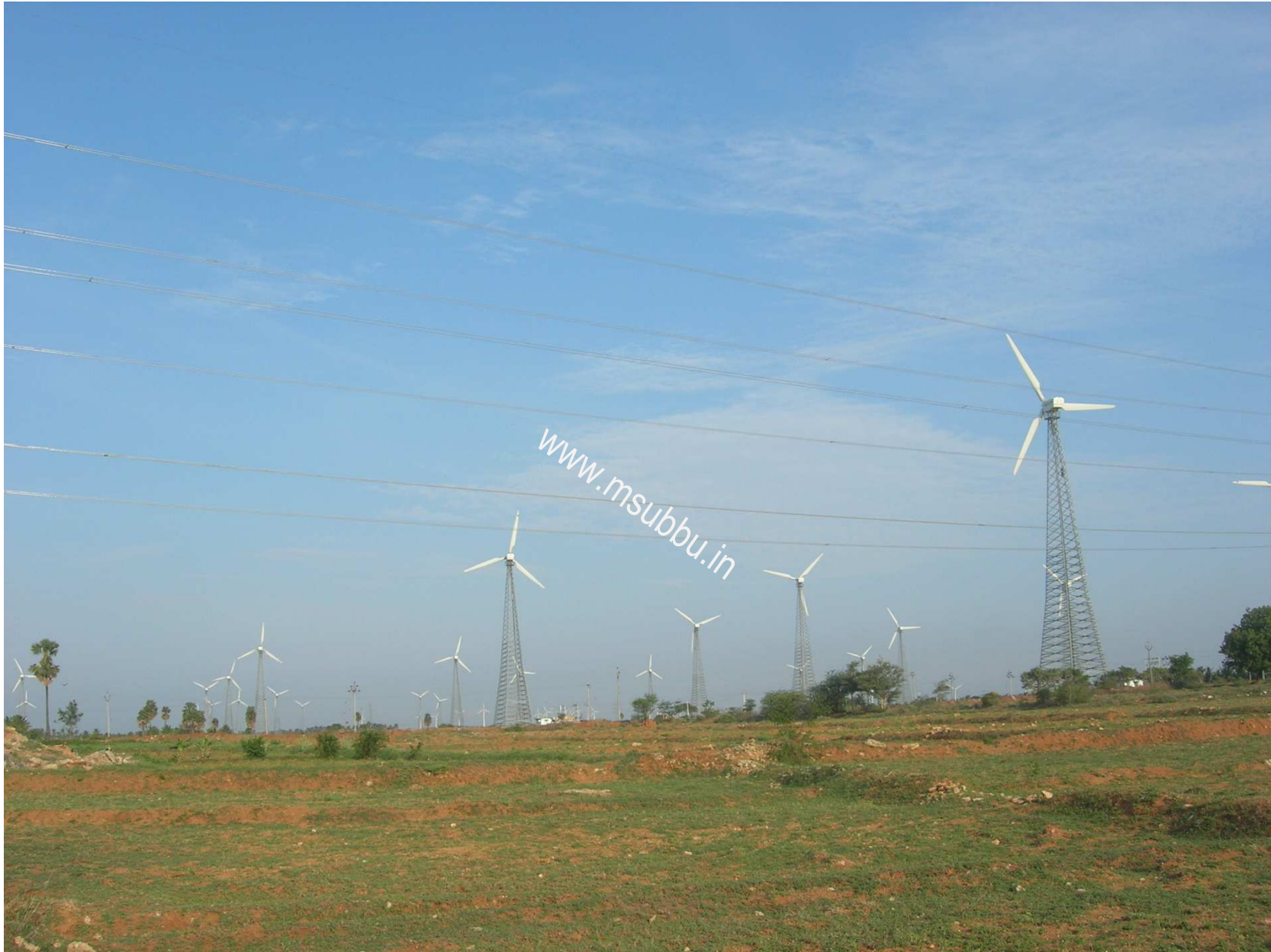
Wind turbines in Udumalpet (Tamil Nadu)
