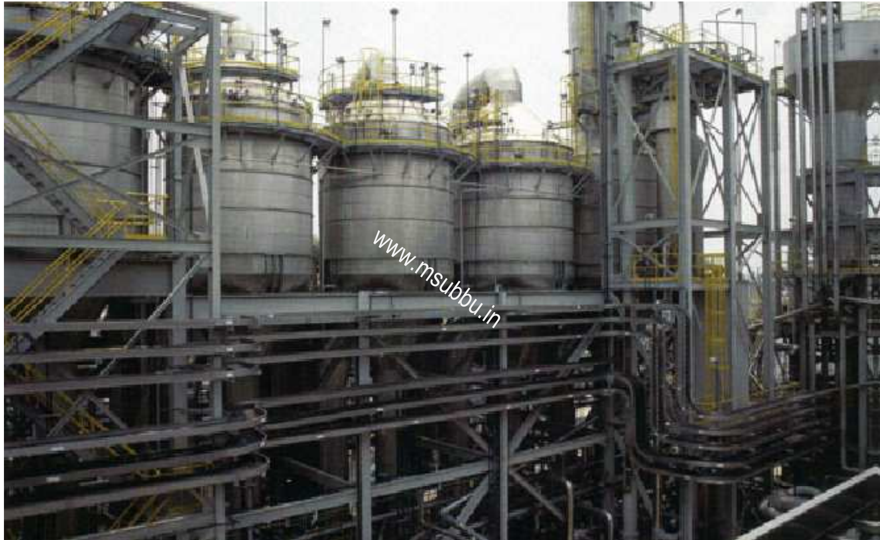
Quintuple-Effect, Forced-Circulation NaCl Evaporator
